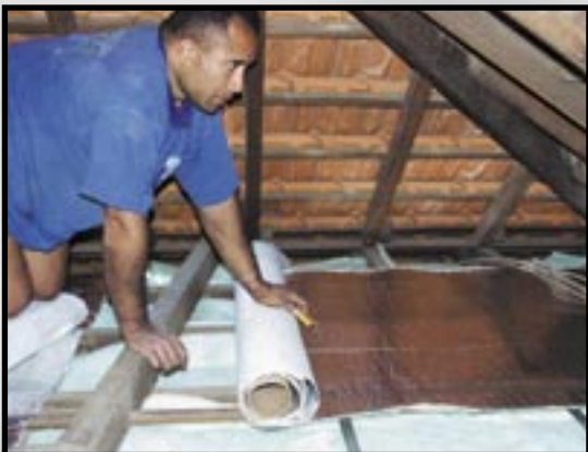
Wavebar ® in roofs shuts out overhead aircraft noise
